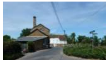
Overhead wires in vicinity of the mill
