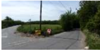
Cluttered signage on roads close to the mills
